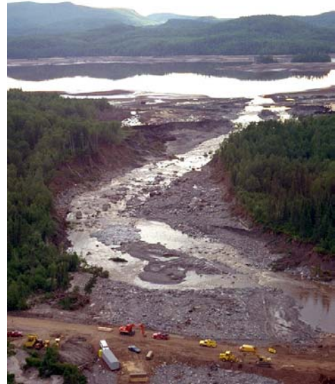
(A) Lake Ha!Ha! Canada, July 1996 - Looking upstream at the breached dam (Courtesy of Natural Resources Canada)
